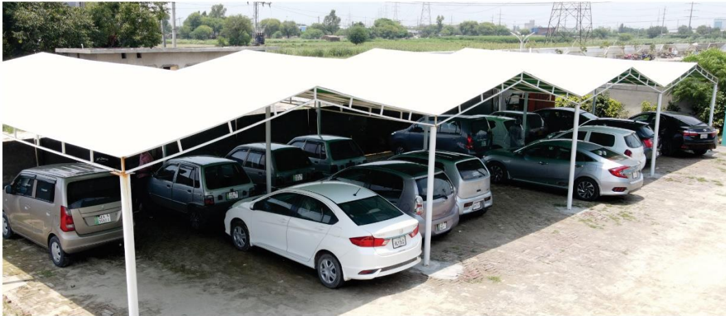
Spacious Car Parking Facility
